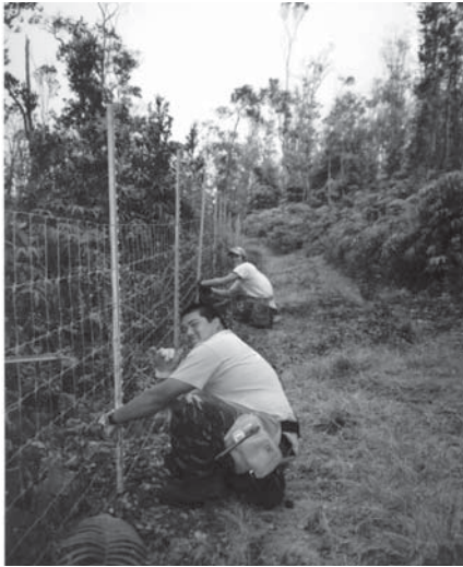
Building fence at Kipahoe NAR
